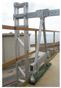
The overhang parapet clamp is mounted on the front member of a FIXAPOUTRE suspension beam placed horizontally. The beam must be installed first.
