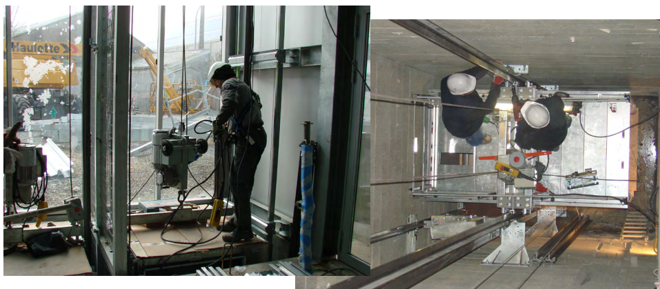
Securichute anti-fall device (mandatory when lifting people) with wire-cable claws and counterweight*.
